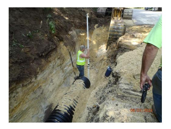
As they were installing the storm sewer up Hill Street, they encountered rock excavation for approximately 60 ft. The picture above shows some of the rock (sandstone) on the edge of the trench.
